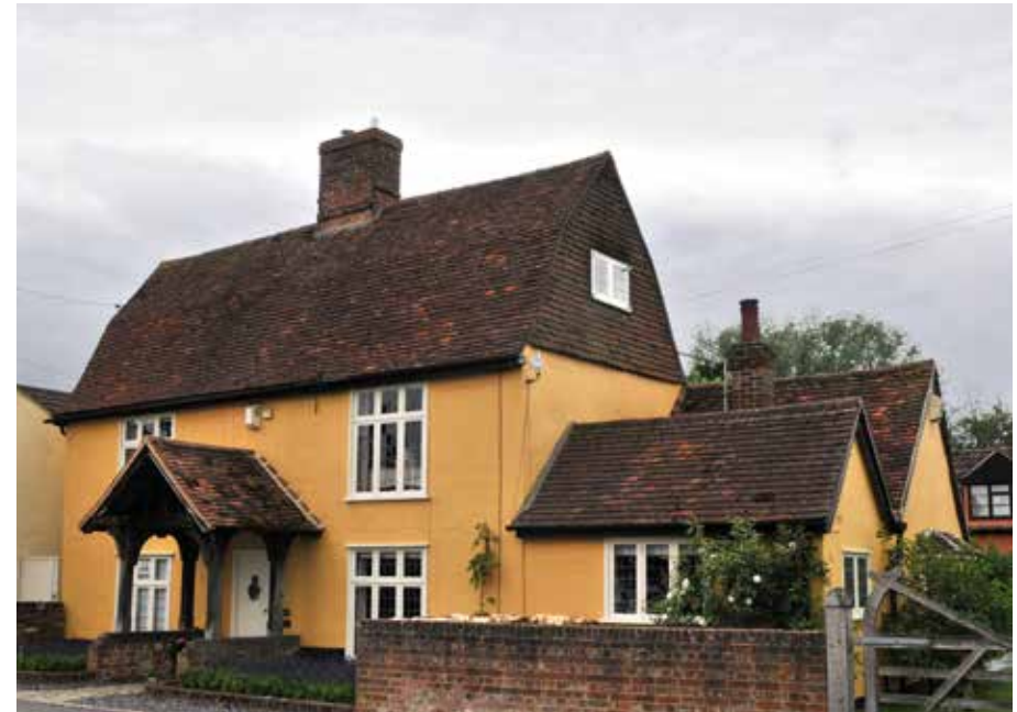
Grade-II listed house with clay tile gambrel roof, gable weatherboarding, leaded windows, and timber-framed gabled porch.
