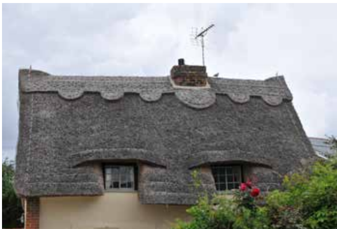
Figure 53: Gable thatched roof with chimney stack and dormers.
