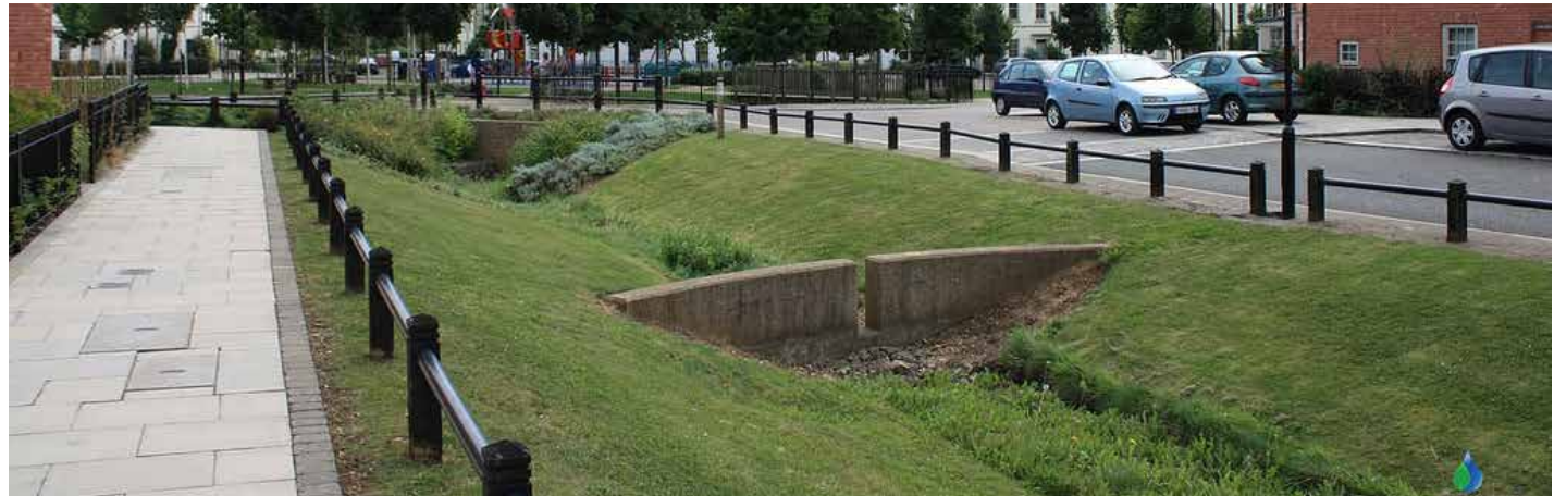
Figure 81: Attenuation swale with check dam (@ Susdrain).
