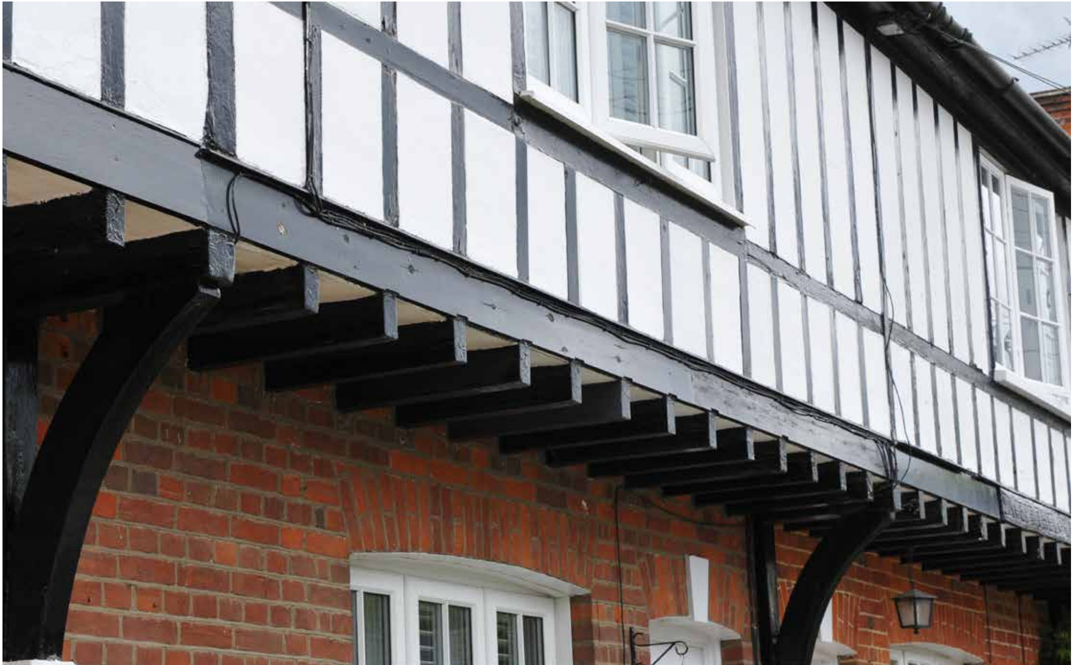
Figure 91: Details of a building with a half-timbered jettied upper storey, Stambourne Road.
