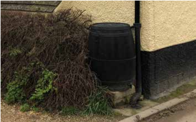
Figure 74: Examples of water butts used for rainwater harvesting in Reach, Cambridgeshire.
