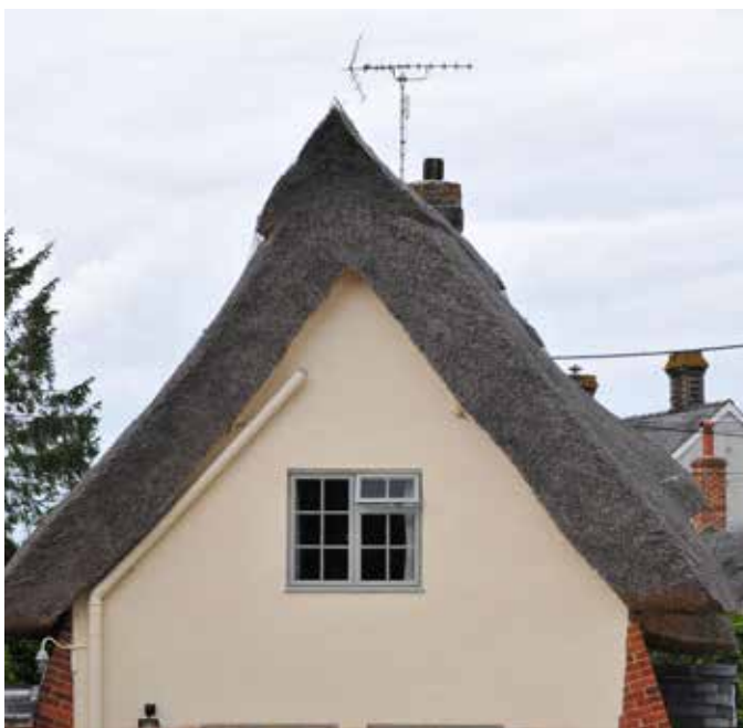
Side elevation showing a recently restored thatched roof and red brick buttresses supporting the front elevation
