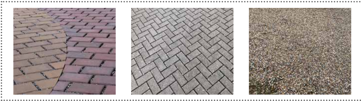
Figure 78: Examples of permeable paving treatments: unbound clay pavers (left), precast concrete setts (centre), and gravel (right).
